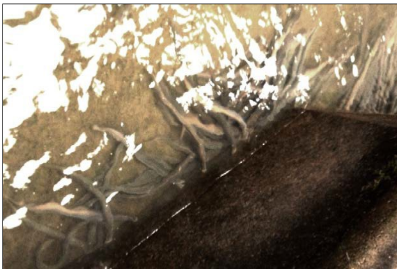
Figure 11. Adult lamprey congregate in the AWS channel of the BON Cascades Island Ladder. Photograph was taken during a mid-season dewatering event in 2013. In winter 2013-14, USACE intends to install 0.75-inch opening picket leads downstream of the channel to prevent lamprey from accessing this dead end channel.
