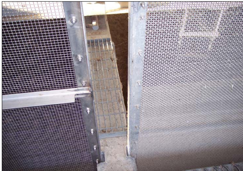
Figure 20. Screening developed for juvenile lamprey separation, (shown in 2009 test at MCN) in dam bypass systems. The screen on the left is the new 6.5 mm spacing that has been adopted at all of the facilities with transport raceways.
