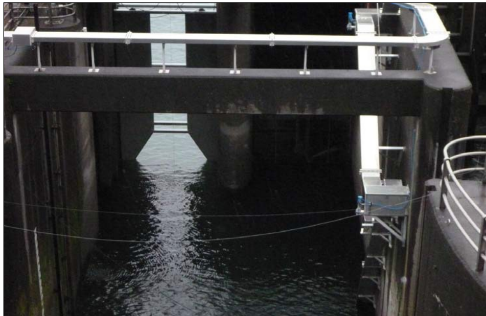
Figure 13. The large turning pool in lower Cascades Island Ladder and in similar ladders may cause migration delays for Pacific lamprey. The new Cascades Island entrance LPS (right) diverts some lamprey out of the main ladder and into an alternative system.
