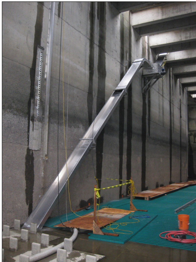
Figure 7. Photo of John Day North Ladder entrance LPS, which was installed during the 2012-2013 winter maintenance period as part of the broader entrance improvements at this fishway. In operation between 19 July and 10 September, a total of 62 lamprey were collected from the LPS and released above the dam.
